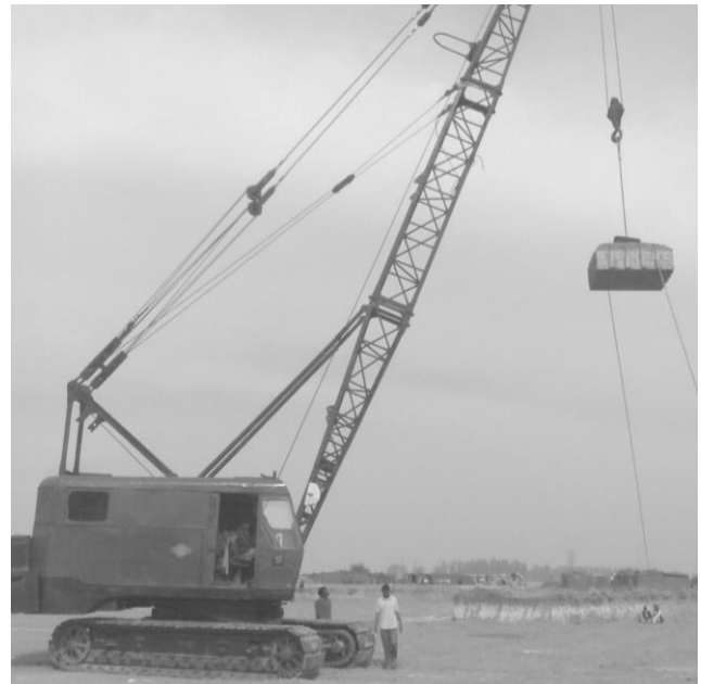
Figure 4. Dynamic Compaction in progress on site
